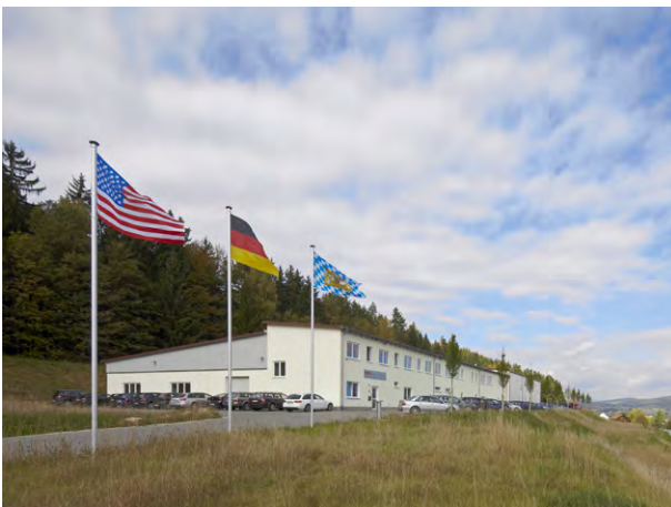
Manufacturing center (Bad Kötzing)
